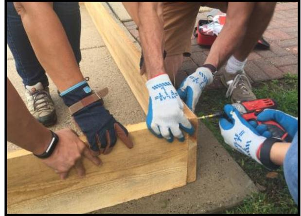
**Step 5: Set the frame into position.** If needed, level the ground under the boards so the lumber makes full contact with the ground all the way around. Avoid gaps between the frame and the ground to prevent soil from leaking out. You may need to use a pick ax, or shovel to dig a small trench. Use a level to ensure the boards are level, this will prevent soil from spilling out over the top during rainstorms.
