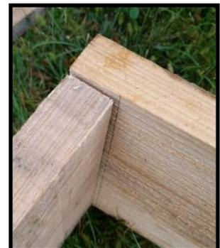
**STEP 4: Build the frame.** Using the star driver bit use the pilot holes as a guide to screw the boards together with the 2.5 inch screws in three places: top, middle, and bottom. Repeat at the remaining 3 corners. Do not attach the cross bracing board yet.
