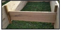
Make the tops of the stakes flush with the top of the bed. **Secure the cross-bracing board to the stakes** with 2 screws for each stake, then secure both outer side boards to the <u>stakes</u>, using 2 screws per side board. You do not need to attach the side boards to the cross-bracing board.
