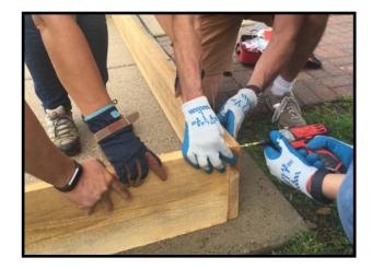
Step 5: Set the frame into position. If needed, level the ground under the boards so the lumber makes full contact with the ground all the way around. Avoid gaps between the frame and the ground to prevent soil from leaking out. You may need to use a pick ax, or shovel to dig a small trench. Use a level to ensure the boards are level, this will prevent soil from spilling out over the top during rainstorms.
